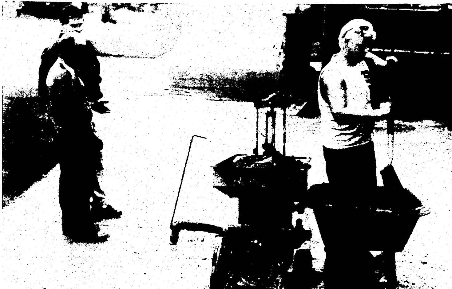
Jim Reid, front left, and Jim Jameson inspect a driveway being lifted by Jim Hixson. As much as five cubic yards of slurry may have to be pumped
