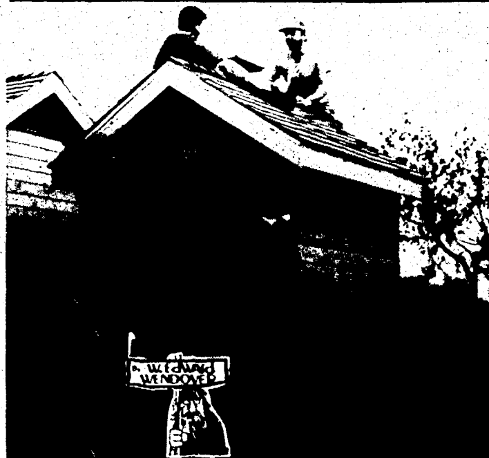
The finishing touches to the Geer School outhouse are added by Chuck Hamlin and Gregg Dunphy of Vipperman Building. (Crier photo by W. Edward Wendover)
