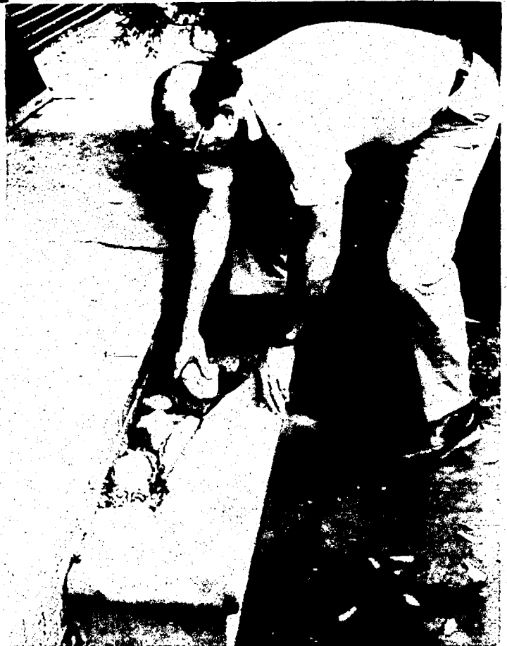
Brian P. Murphy, a safety consultant, with Basic Ideas, Inc. inspects a deteriorating step that was not properly maintained. (Crier photo by Ken Voyles)
