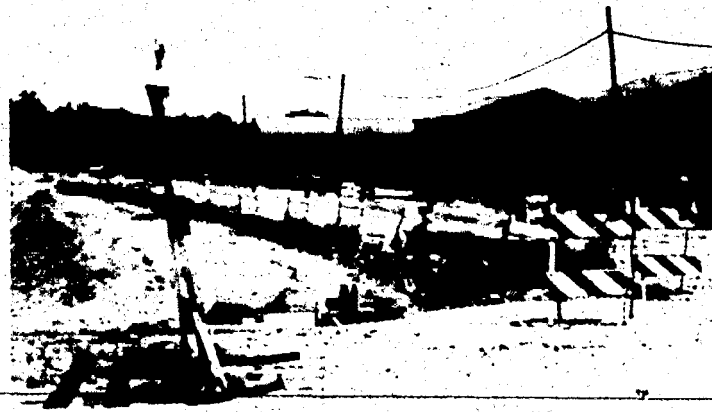
One of the many paving projects underway this summer includes this stretch of Warren Road in Canton. (Crier photo by Kelly Sauter-Dobson)
