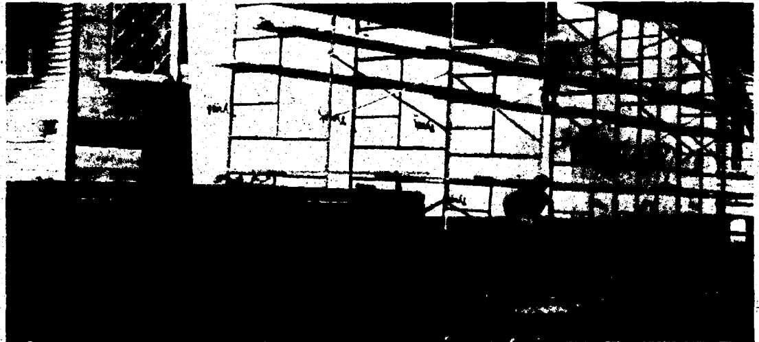
Workers begin the long process of renovating the historic Wilcox House in downtown Plymouth. The Plymouth Planning Commission recently approved a PUD for the project. (Crier photo by Chris Farina)
