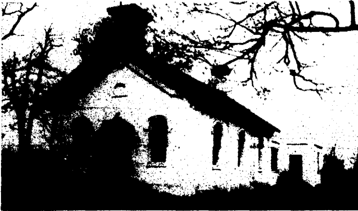
Cherry Hill School in Canton under renovation. (Crier photo by Chris Farina)
