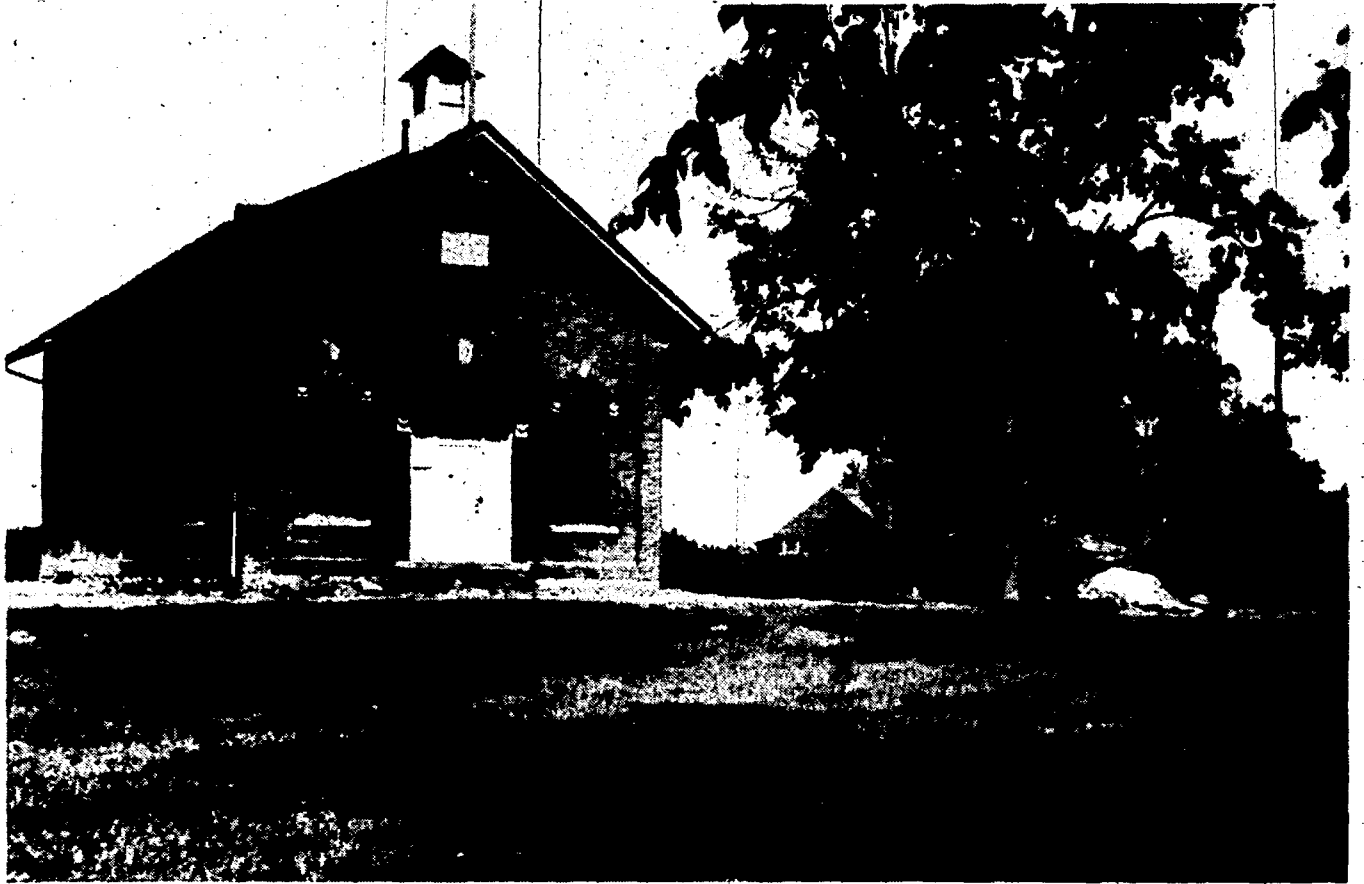
Geer school restoration work continues. At right, is a pile of rubble from work done earlier. The restoration
