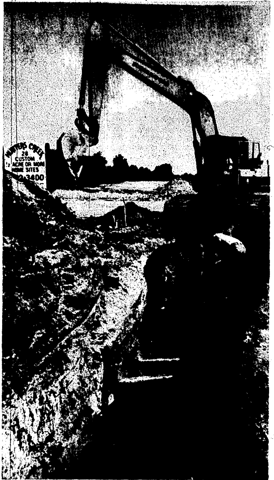
Work continues along Powell Road as development projects lead to the paving of Plymouth Township roads. (Crier photo)
