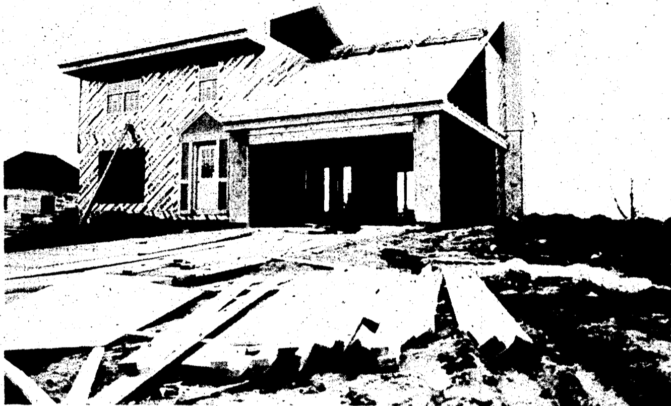
New homes being built are a familiar site in Canton. This house is part of the latest Sunflower subdivision project in Canton. (Crier photo by Dan Ness)
