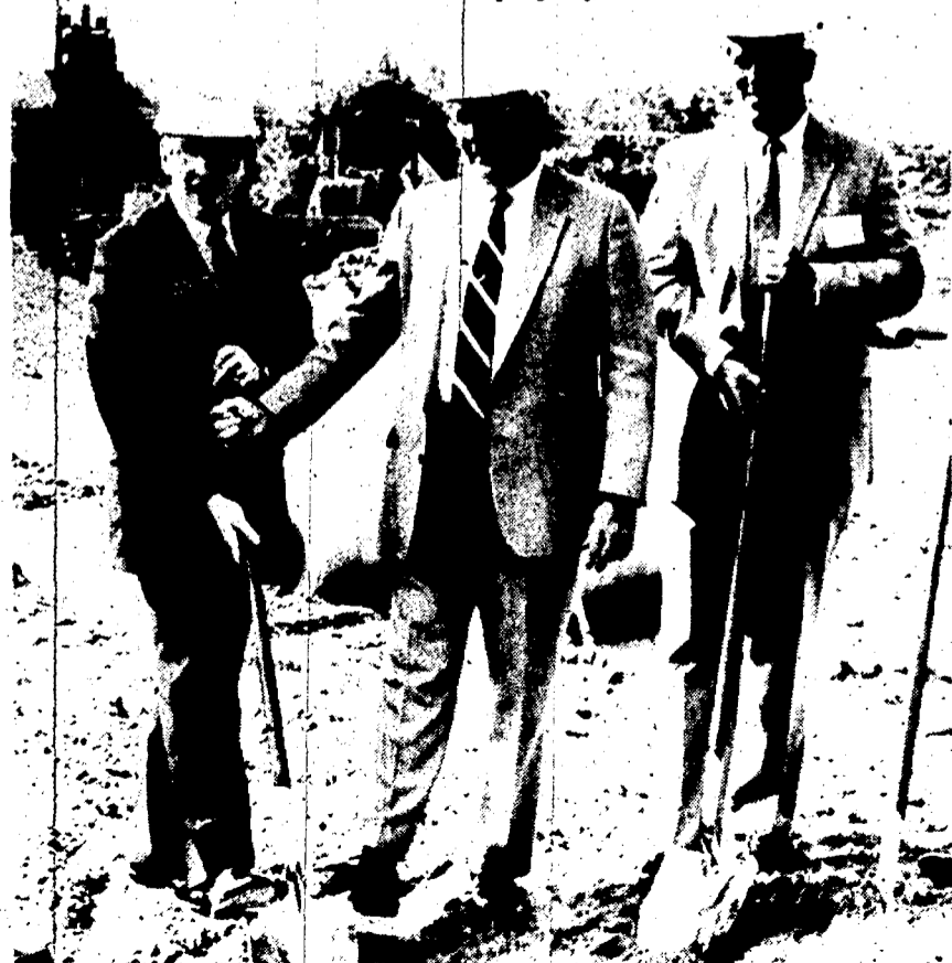
Schoolcraft Board President Mike Burley, college President Richard McDowell (center) and a Duke Associate, partner dig in during last week's groundbreaking. (Crier photo by Ken Voyles)
