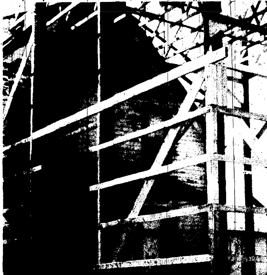
CONSTRUCTION IS UNDERWAY at the site on Union Street. (Crier photo by Rachael Dolson.)
