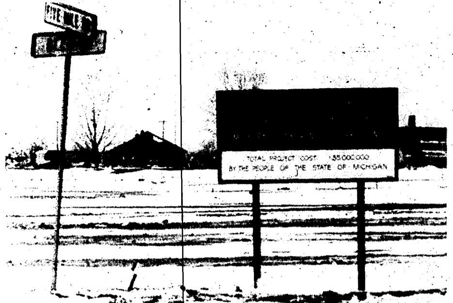
CONSTRUCTION OF the $35 million new state prison has been halted by cash flow concerns. The ground has already been cleared for the planned prison at Beck and Five Mile roads. (Crier photo by Rick Smith)
