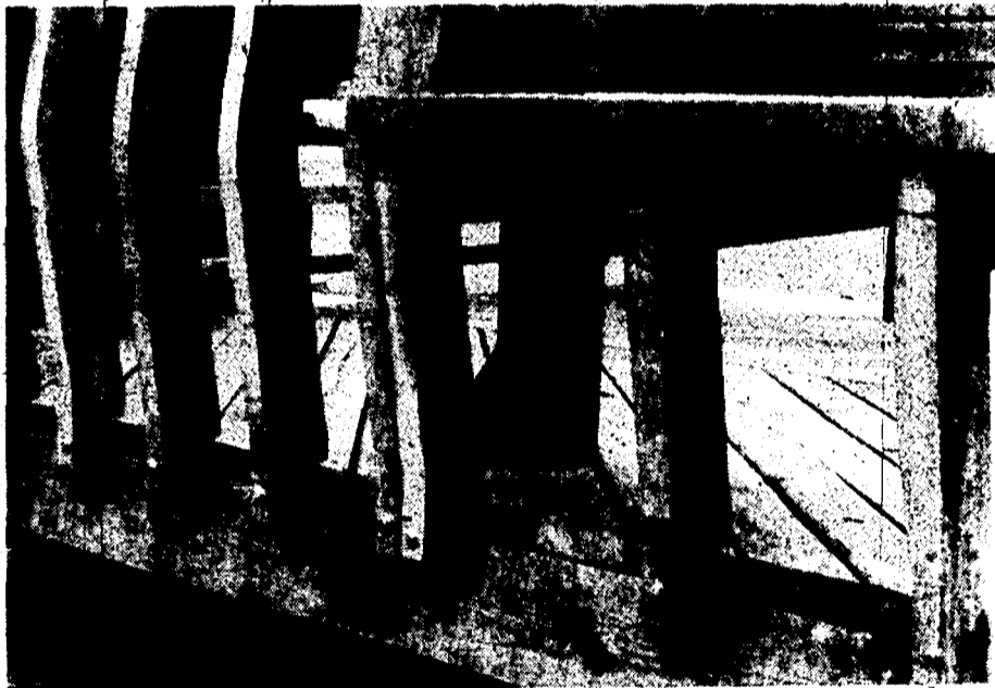
DETAILS of the deck railings show the outboard mounting scheme, which doesn't encroach on the floor space of the deck, and the bolts that secure railing supports to the deck. Up-to-date deck designs rarely rely on railing supports for overall strength of the deck: structural support is all underneath. Other details include curved railing supports, which can be sawed in half to make bench supports. (Crier photo by Dan Bodene)
