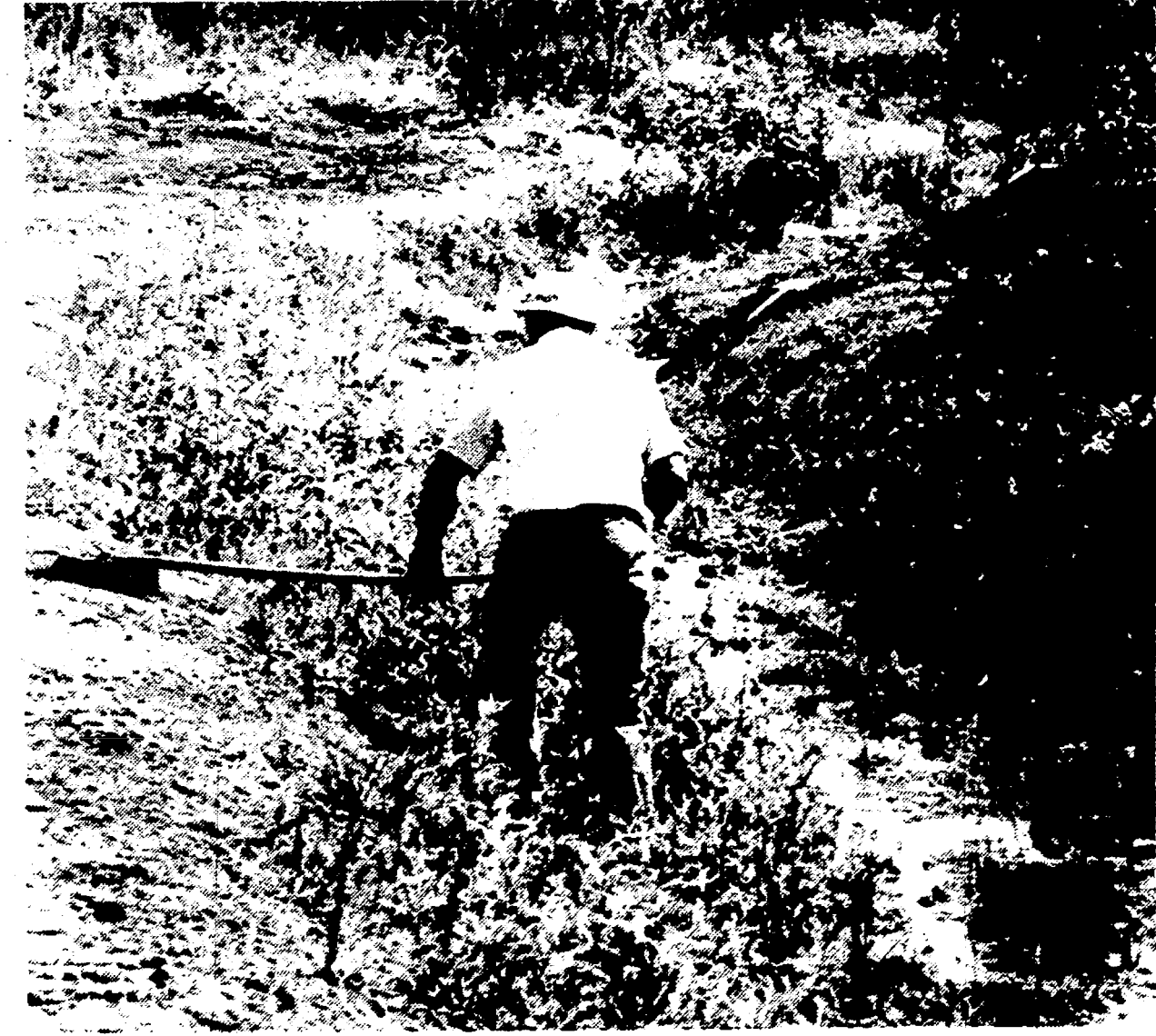
ONE OF THE LAST HURDLES for the new Oakwood Center was improving the drain along its northern edge. Final approval for the work is still pending.
