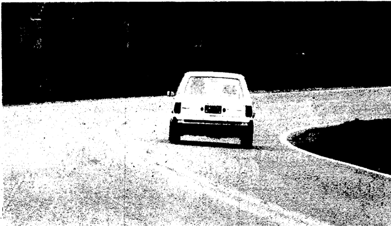
IN THE TOP photo is North Territorial Road looking east at the first of two sharp curves. Note the rise in the road and sharpness of the turn. The bottom photo shows the west curve looking westward. Note the semi blocked speed limit sign, the hard-to-see curve direction markers and the steep rise just before the curve itself, which effectively blocks a drivers vision upon entering the curve. (Crier photos by Robert Cameron)
