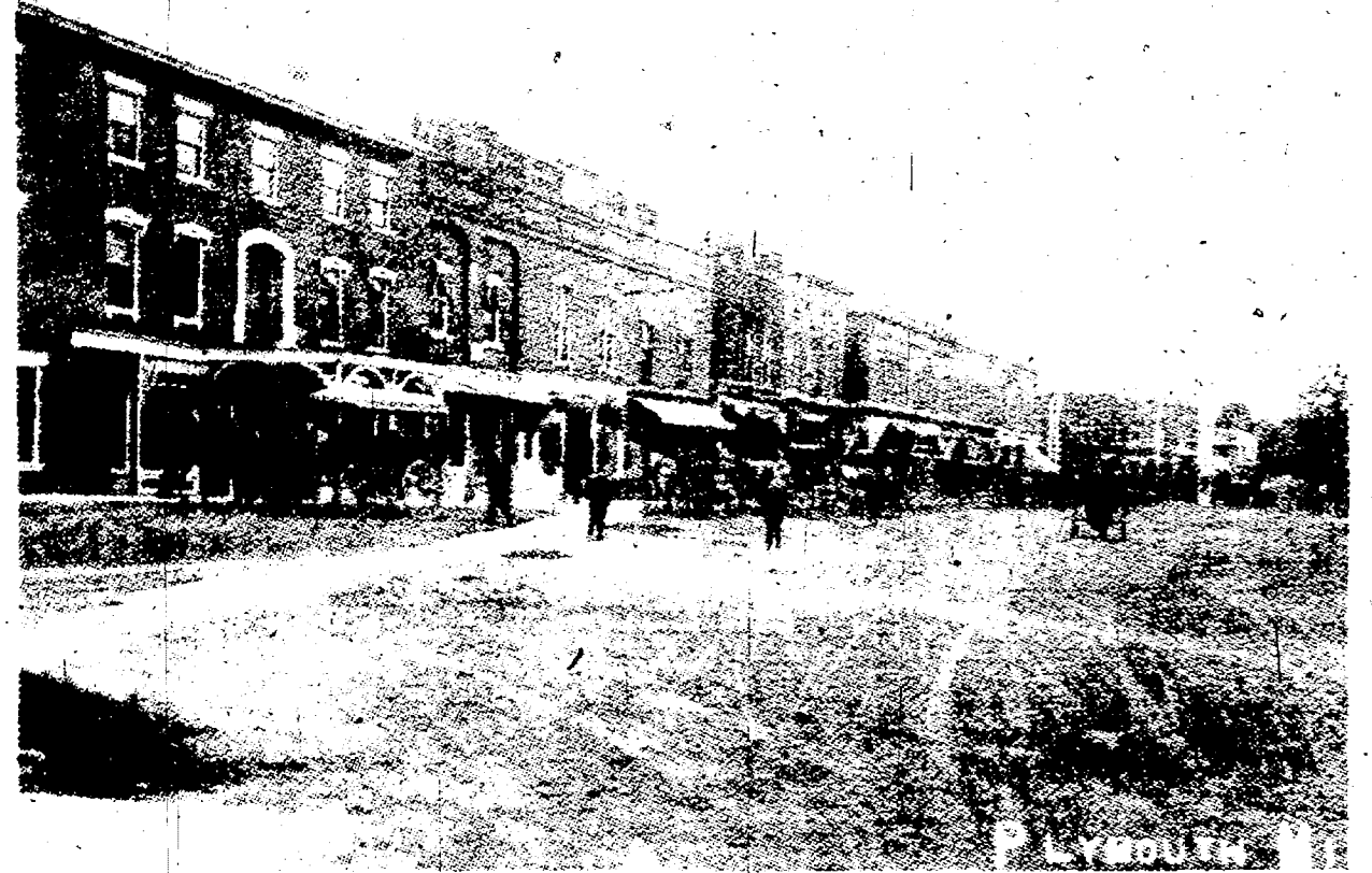
AFTER THE 1893 FIRE, the "Phoenix Block" on Main Street had already risen from the ashes as shown in this undated photo. Some of the structures will remain, such as the old Conner building at the corner of Main and Penniman, shown at the far right. (Photo courtesy Sam Hudson' "Pictures of Plymouth, Past and Present")
