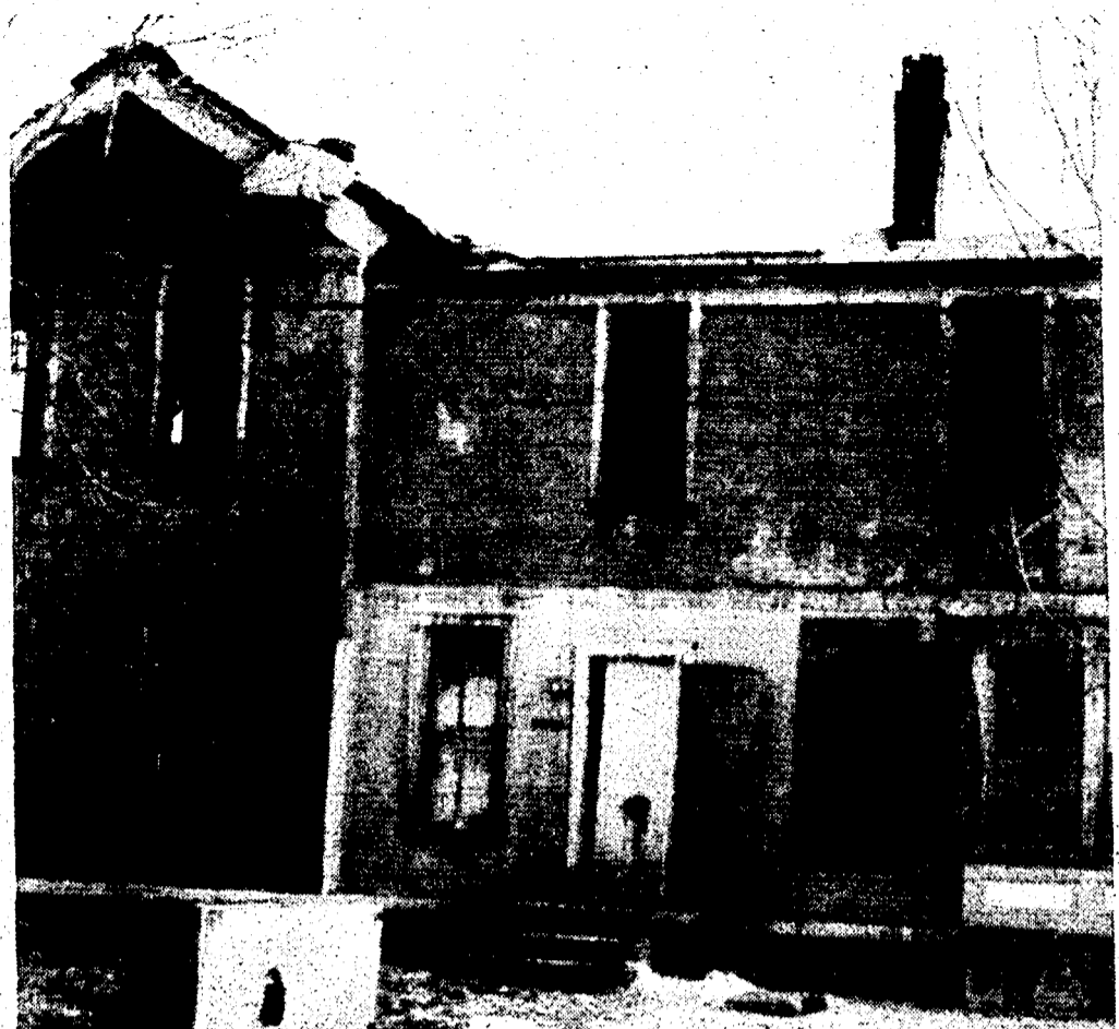
NEARLY DESTROYED by the fire on Christmas Eve, the Pitts home in Canton was further ravaged by water and smoke damage. Until the family can make other living arrangements, they will be staying with friends in Garden City. (Crier photo by Robert Cameron)
