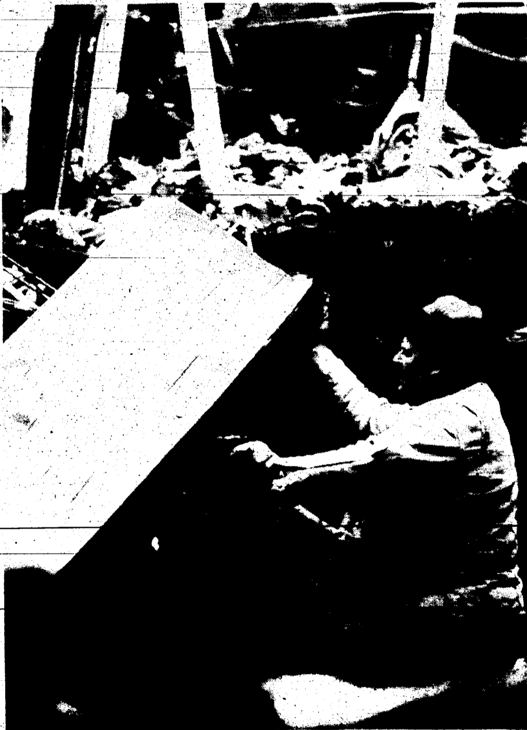
SEARCHING THROUGH the burnt out rubble in the Penniman Avenue Shop building Monday, Lt. Henry Berghoff looks for clues to the Feb. 16 arson and for valuables remaining from the shops. Police and fire officials have said that demolition of the building must begin before parts of the building, ruled unsafe by City Engineer Ken West, can be searched. (Crier photo by Robert Cameron)
