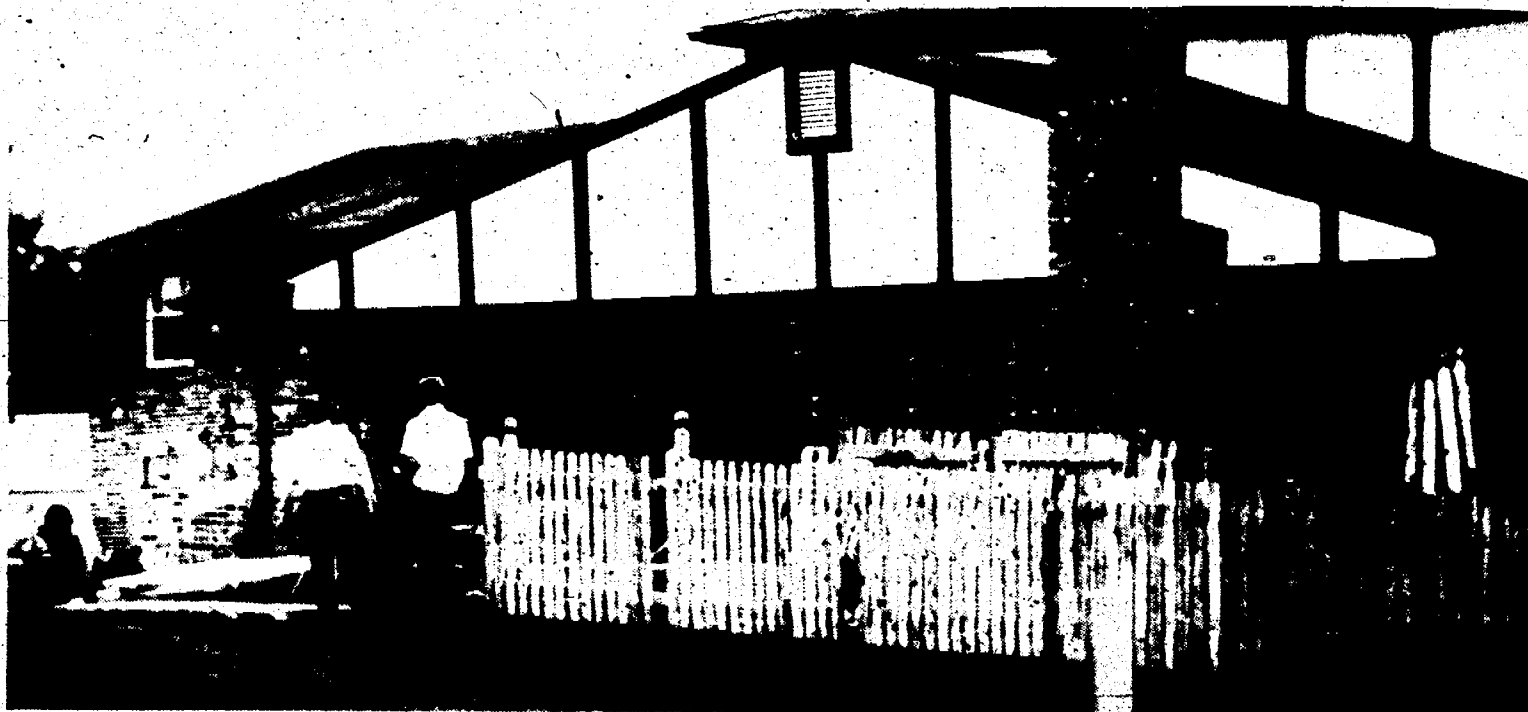
A PETITION PROTESTING the construction of the fence above was signed by about 75 per cent of the homeowners or their spouses in the Quail Hollow subdivision, said Diane Toelle, a neighbor. The fence, put up by Wayne Shpakoff, borders on many other lots in the neighborhood and creates an eyesore, neighbors said.
