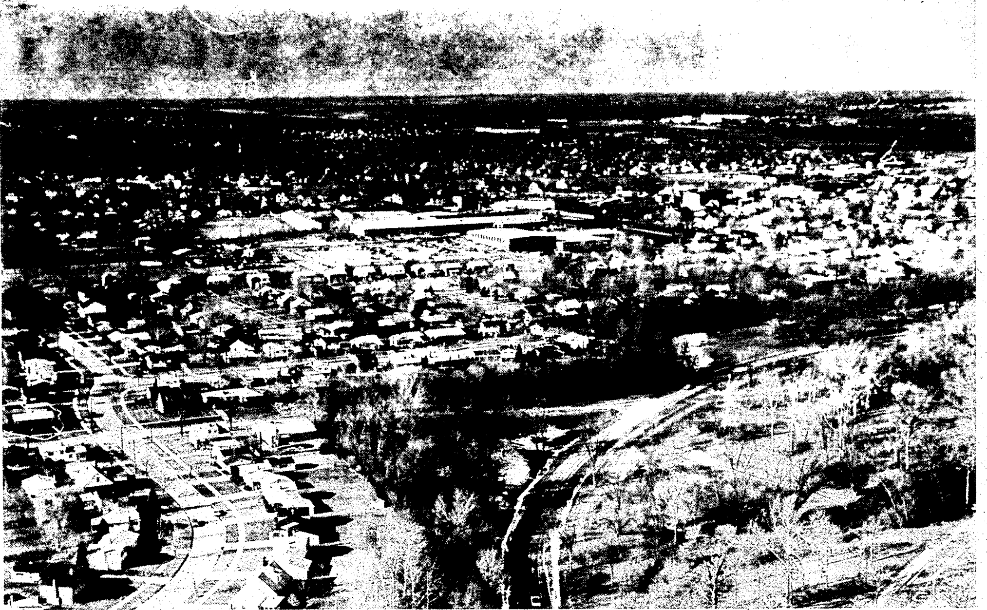
GROWTH in Plymouth Township spurted ahead in 1978 and is expected by some to increase even faster in the future — much like Canton's growth — when the westward extension of sewers is completed. Above is the township and city
