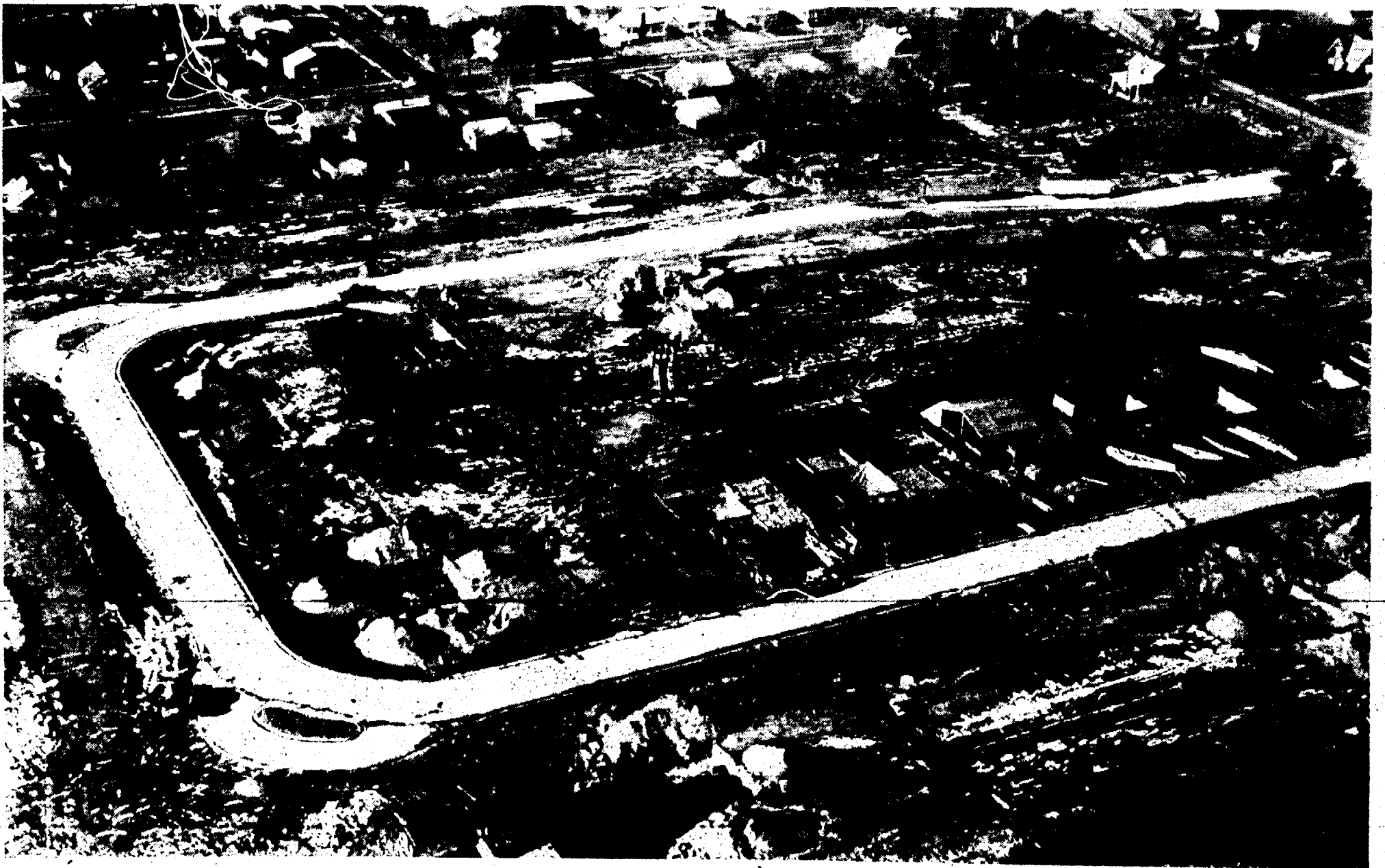
looking westward while below is the street and foundations of one of the last new subdivisions going in on the eastern side of the township. (Crier photos by Bill Bresler, Flight Service by Hi-Lift Helicopters.)
