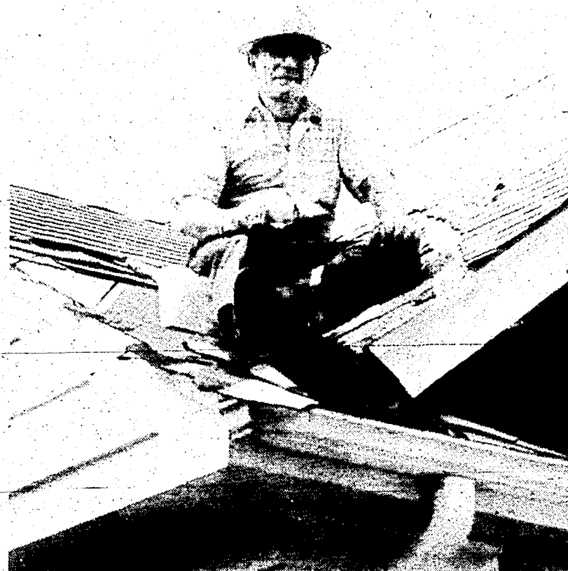
PAUL SANDERS, a 25-year veteran on the City of Plymouth Fire Department, along with other city firefighters, came to the aid of Dan Fowler, a volunteer at the department, by helping repair his roof. Fowler, who was injured, when he fell off a ladder, was unable to finish the roof. (Crier photo by Phyllis Redfern.)
