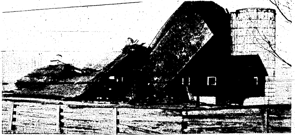
A TIME-RAVAGED barn on North Territorial Road west of Curtis, in the process of collapse, finally caved in. (Crier photo by Hank Meijer.)
