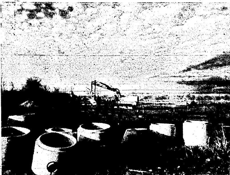
AN ACCIDENT Wednesday killed a construction worker at this subdivision site at Sheldon and Palmer in Canton. (Crier photo by Brian Watkins)
