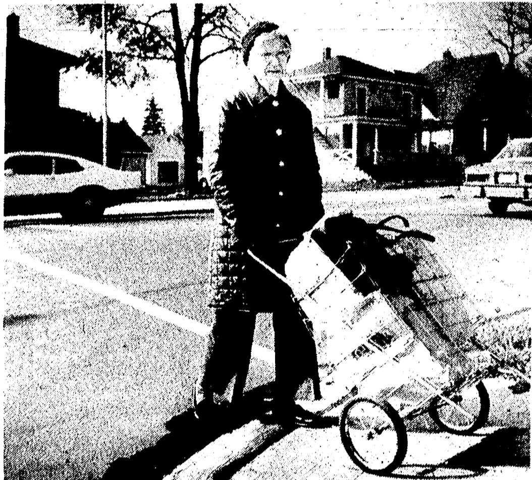
Curb sloping nears completion
