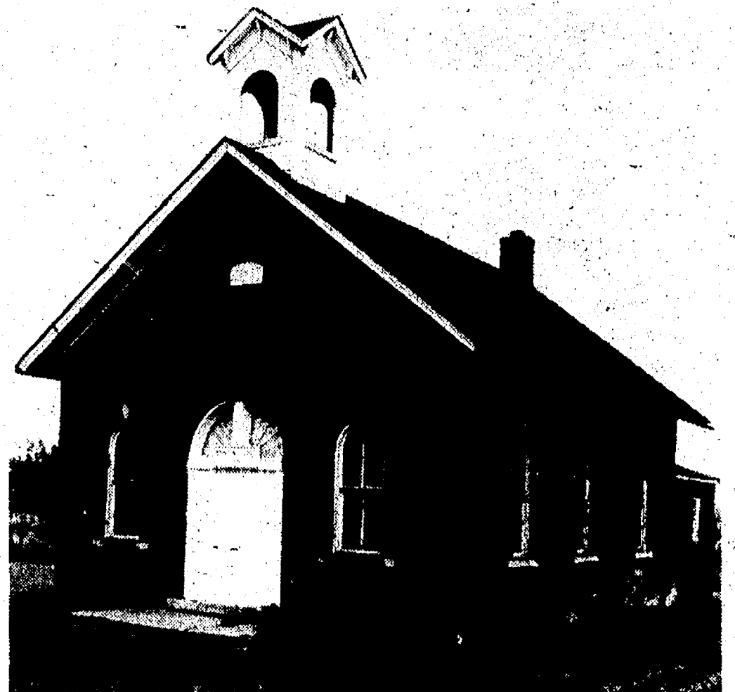
THE OLD BRICK schoolhouse at Canton Center and Proctor may be destined to become the Canton Historical Museum, but that goal is still a long way off.
