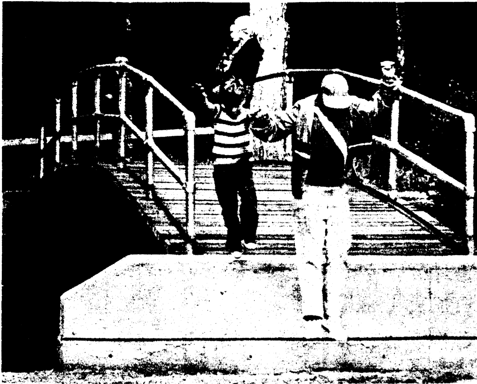
A NEW BRIDGE was completed recently across the Middle Rouge River near a section of Hines Park near Woods Drive in Plymouth Township. According to Wayne County Road Commission spokesman John Kinville, the 65-
