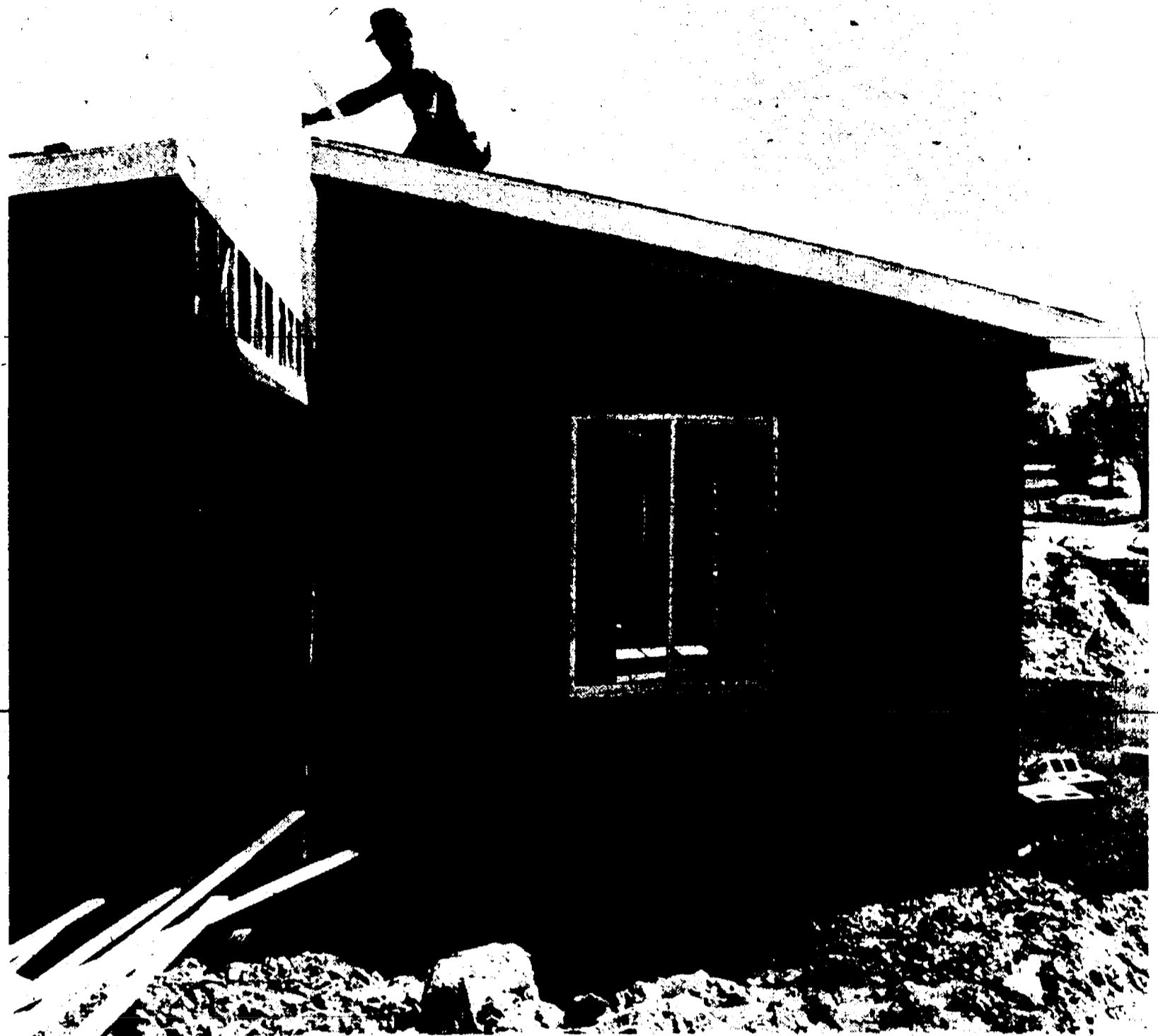
A NEW PREFABRICATED Clubhouse will soon be open to golfers at Plymouth Township's Hilltop Glen Golf Course on Ann Arbor Trail at Powell Road. The two halves of the
